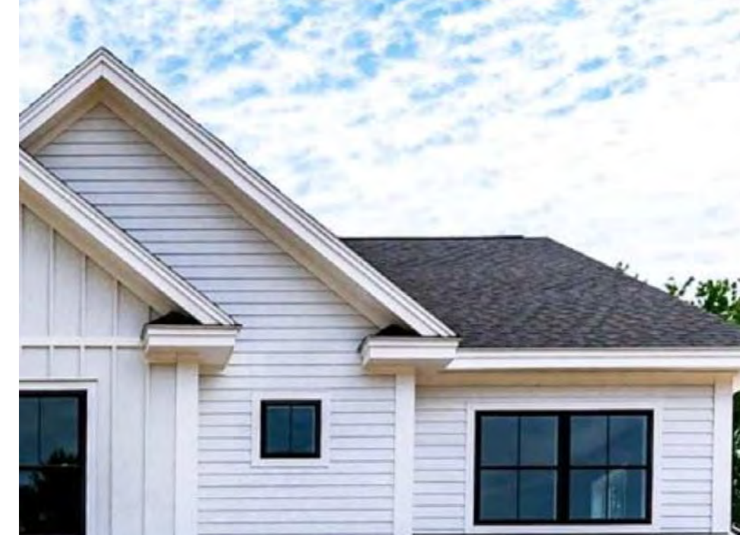
3 HORIZONTAL SIDING MANUFACTURER: HARDI-BOARD COLOR: WHITE FASCIA & WOOD TRIM DETAILS (COLOR: WHITE)
