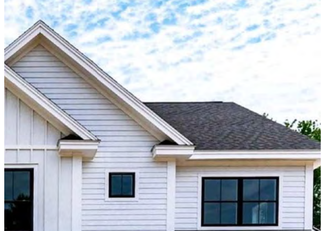
3 HORIZONTAL SIDING MANUFACTURER: HARDI-BOARD COLOR: WHITE FASCIA & WOOD TRIM DETAILS (COLOR: WHITE)
